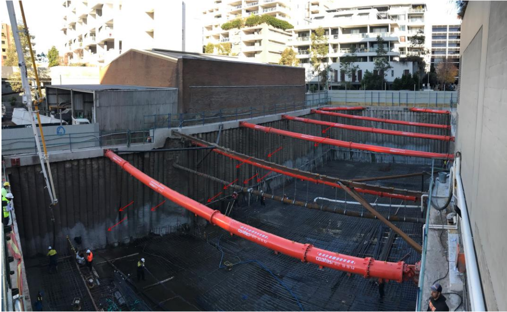
Figure 2: Peak Towers basement construction
